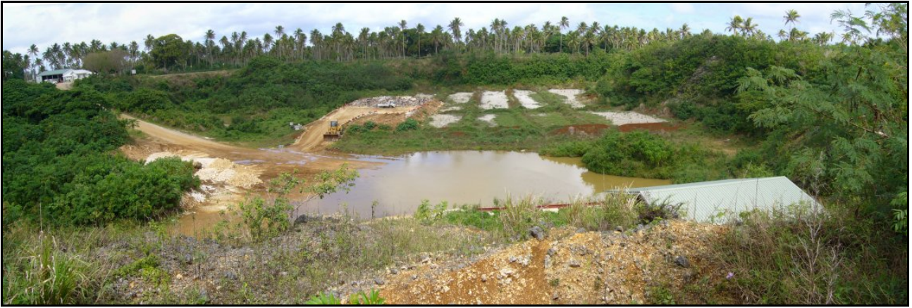
Figure 11 The TWMP located in an abandoned quarry near Vaini. Note the exposed water table at the base of the quarry.
