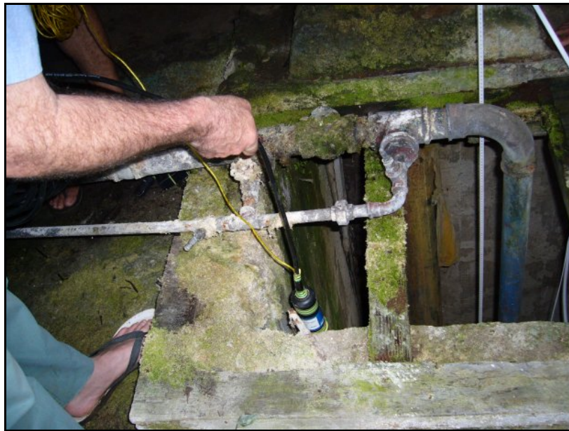
Figure 24 Placing the groundwater logger in Mataki'eua TWN pumping well 117
