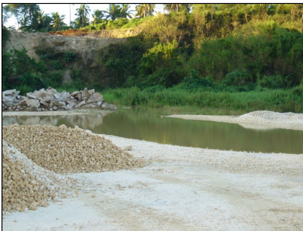
Figure 165 Groundwater exposed at the base of the Kahoua Quarry
