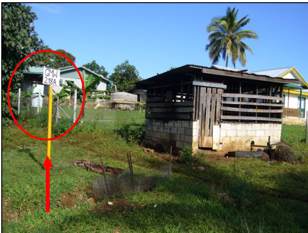
Figure 75 Vaini water supply well, GMW218A, with neighbouring septic tank latrine
