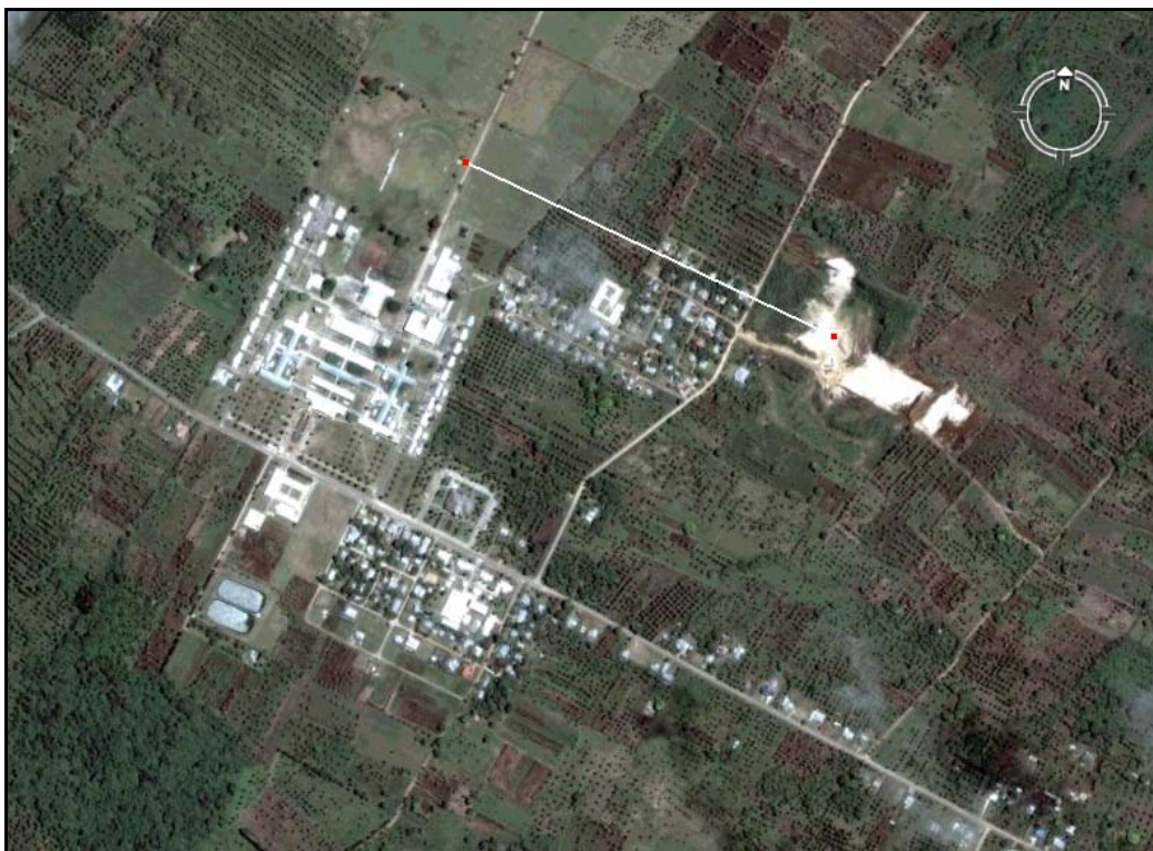
Figure 163 Distance between the Kahoua Quarry and the nearest water supply well at Liahona School. The distance of the line between the red points is 0.7 km.
