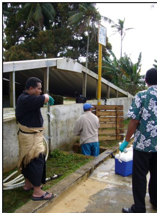
Figure 162 Groundwater monitoring borehole GMW2 beside the sullage drying beds and waste truck wash-down area at the TWMF
